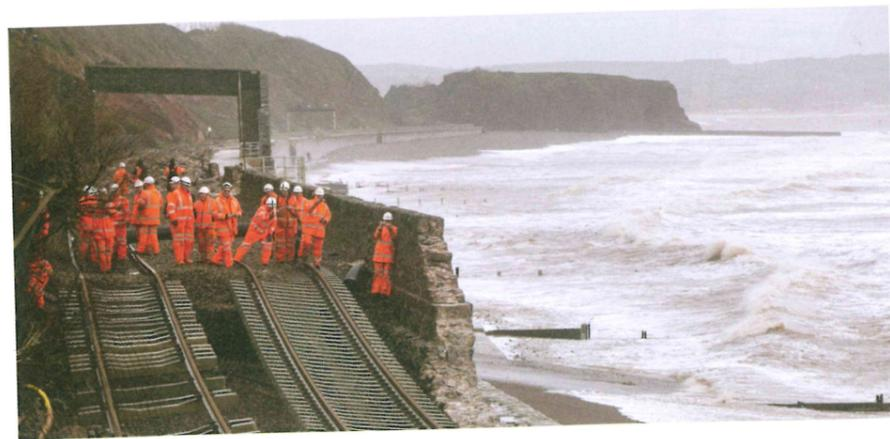
Figure 8.22 Railway workers inspecting the main Exeter to Plymouth railway line at Dawlish which was closed due to parts of it being washed away by the sea on 5 February 2014.
