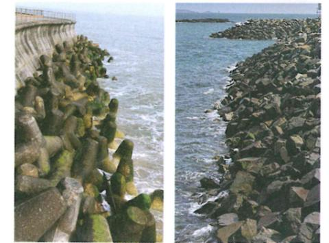
Figure 8.31 Hard engineering techniques – Ventnor to Bonchurch. The photo on the left shows tetrapods; the photo on the right shows rock armour (rip-rap).
